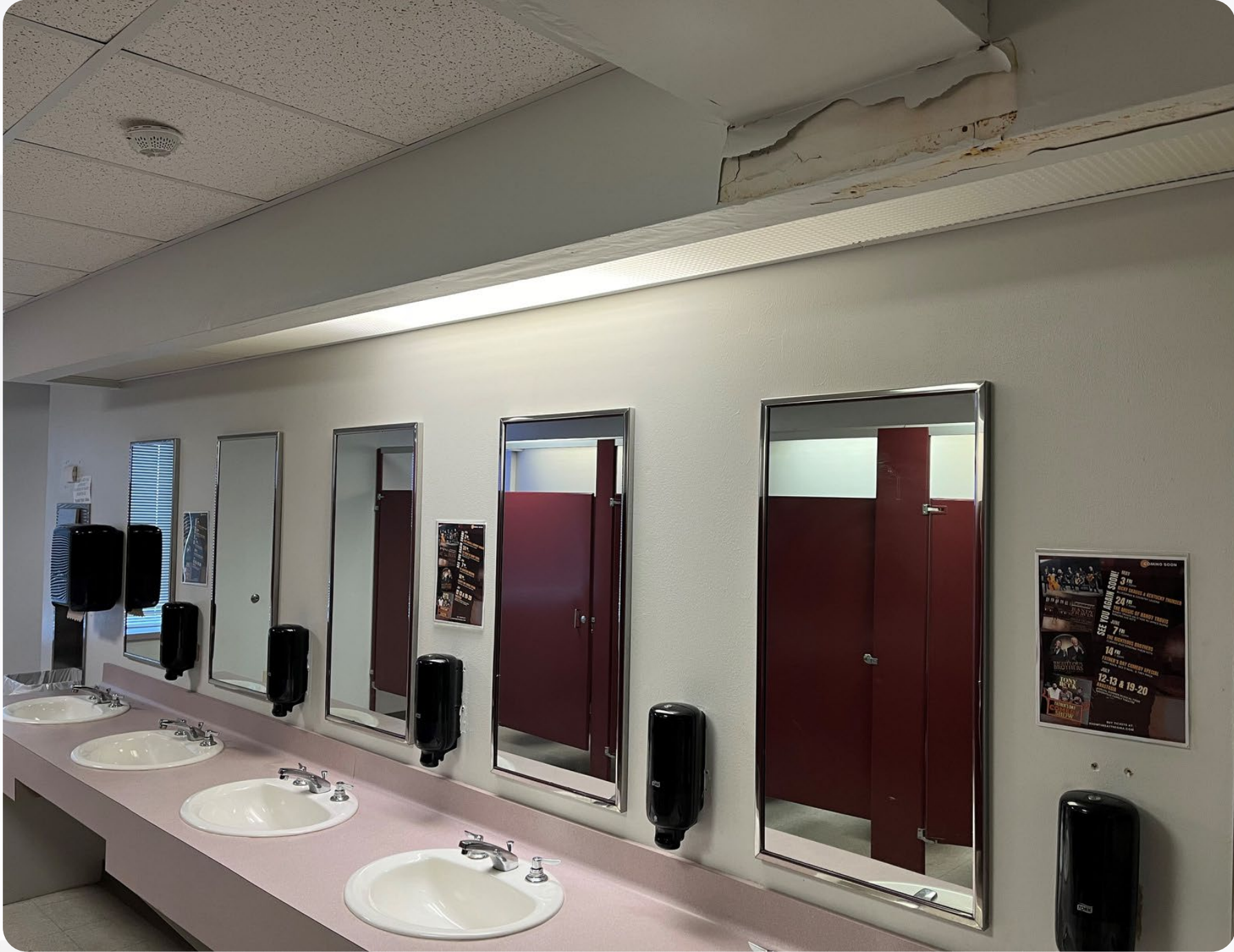
GMA Lobby Bathroom Remodel $175,000
