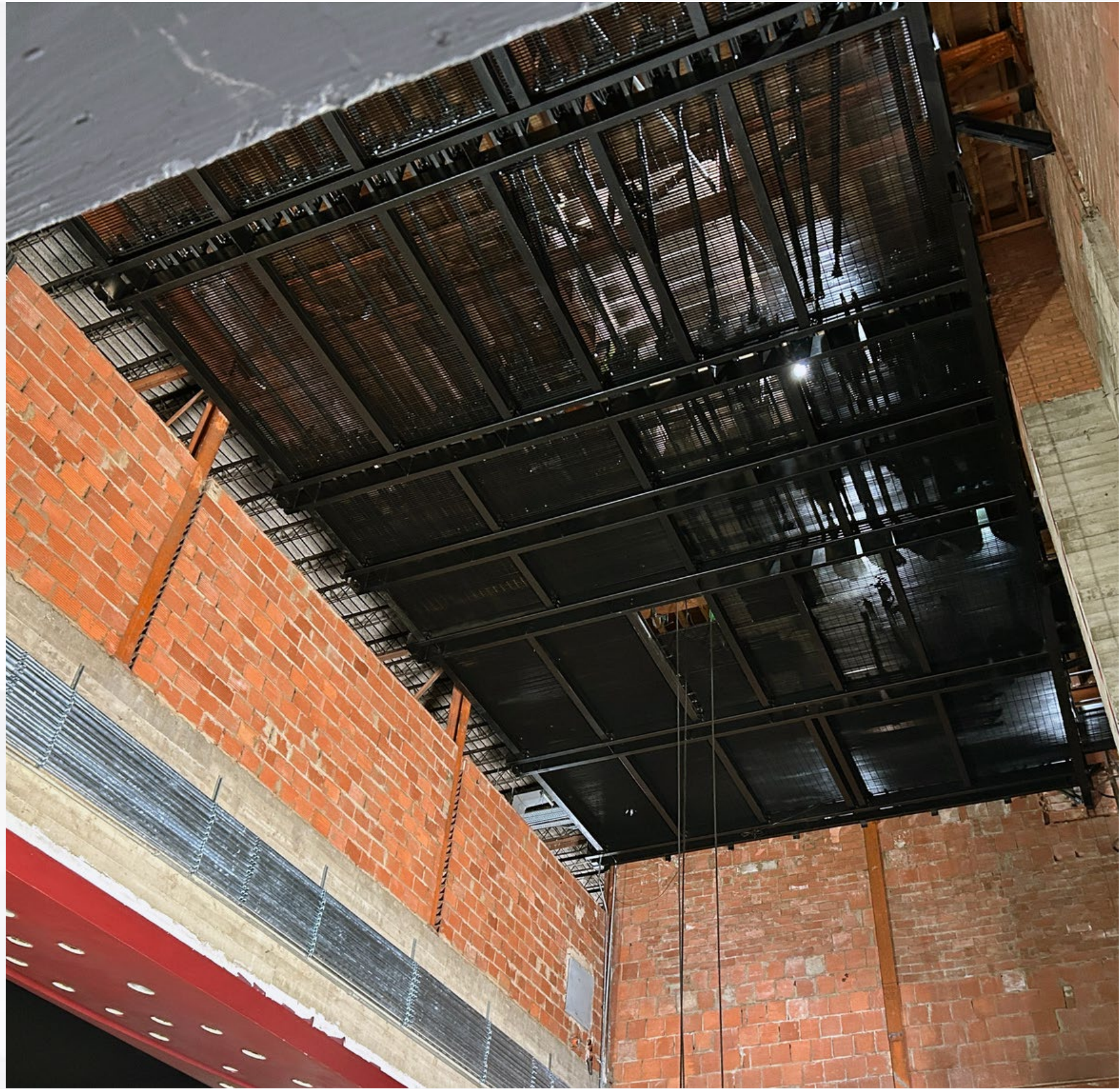
NEW STEEL GRID
