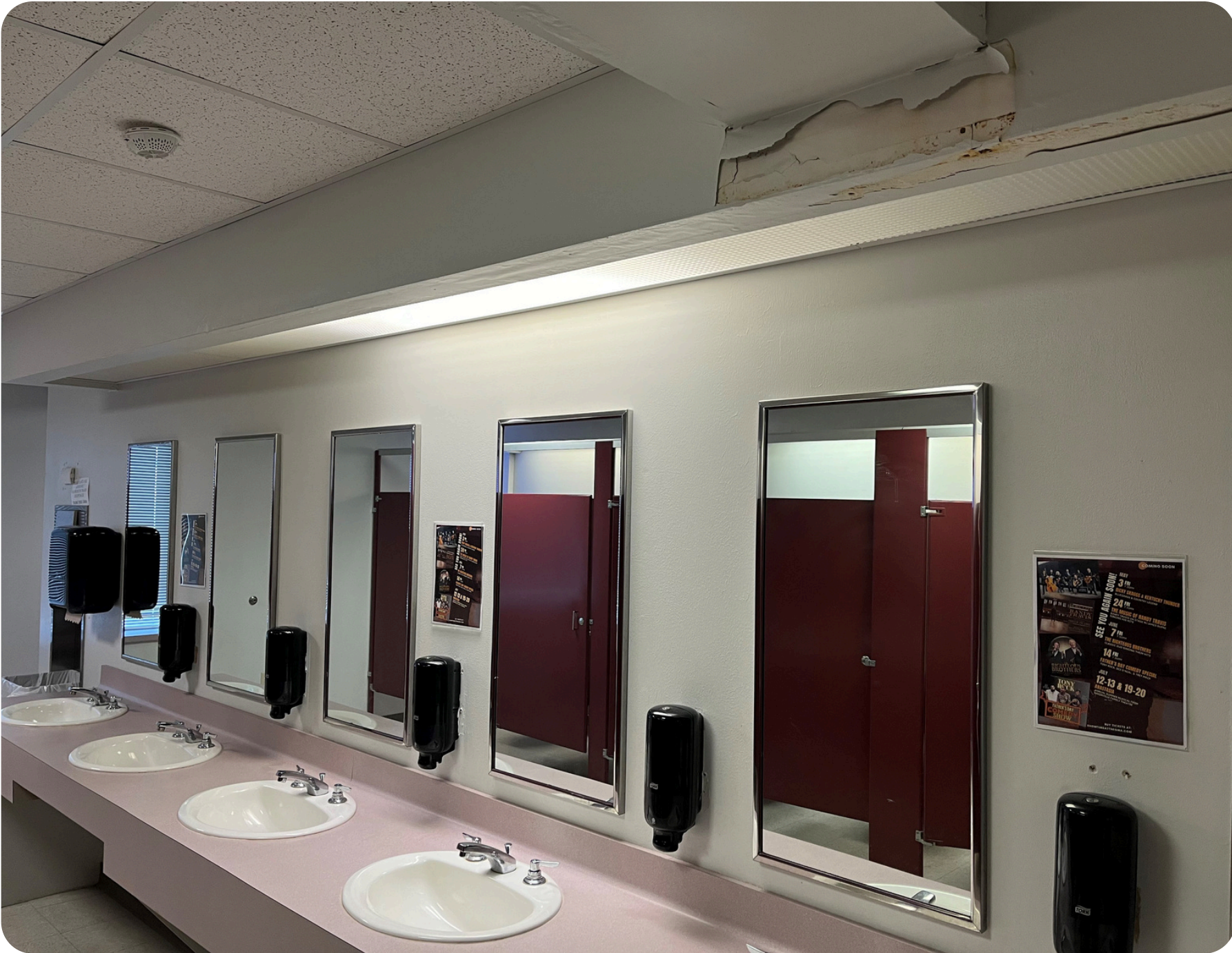
LOBBY BATHROOMS AUGUST INSTALL
